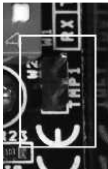
Tamper input additional, in case of absence MUST be closed by jumpers.
